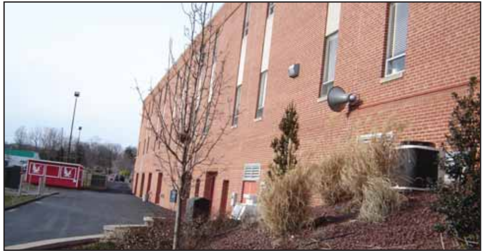
Because the brick school building protrudes past the press box, this fill/delay horn is used to cover the concession and restroom area.
