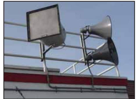
Speakers are mounted on the press box for maximum coverage.
